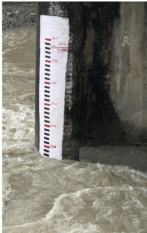
Figure 3.1: Staff Gauge or Manual Gauge at Chel, West Bengal
